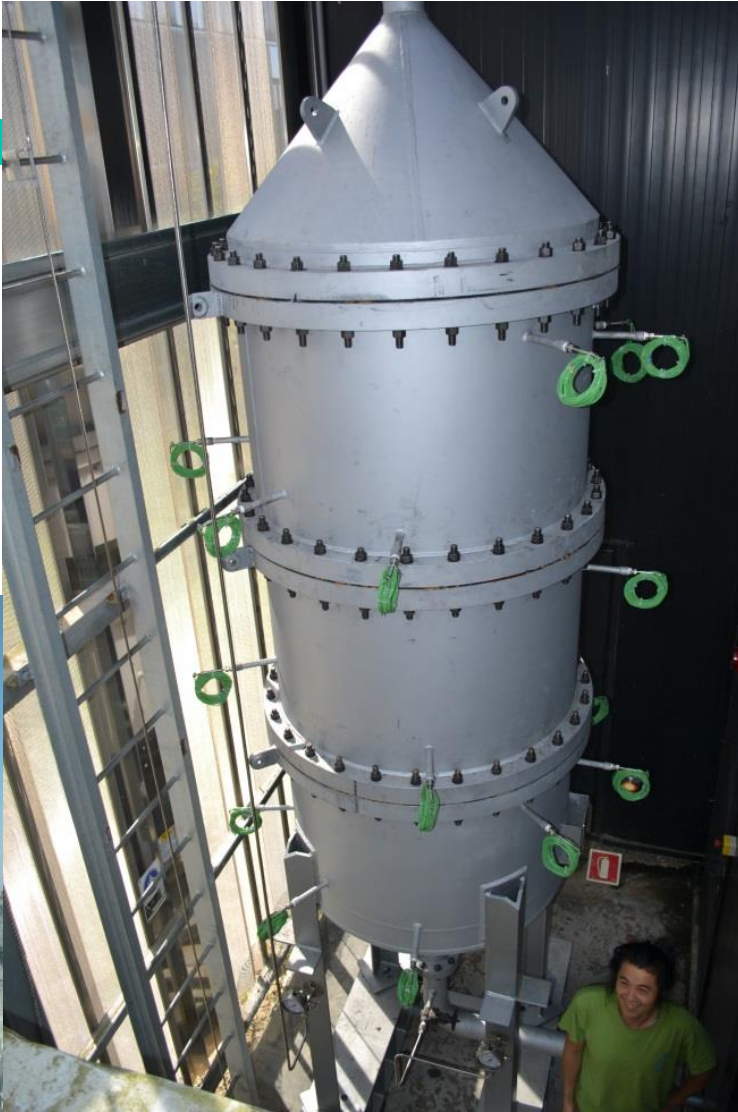
H2020 ORC-PLUS Project 200 kWh t packed bed thermocline ~ 6.5 tons of storage material
