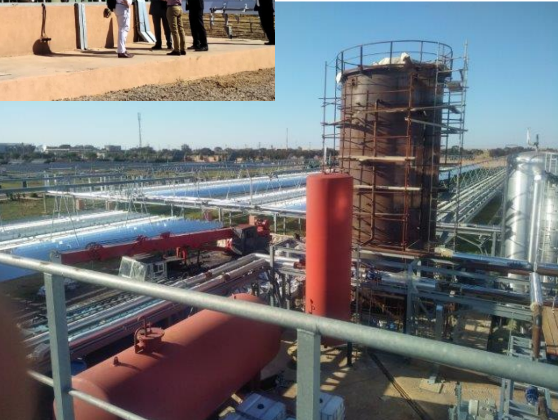
H2020 ORC-PLUS Project 200 kWh t packed bed thermocline ~ 6.5 tons of storage material
